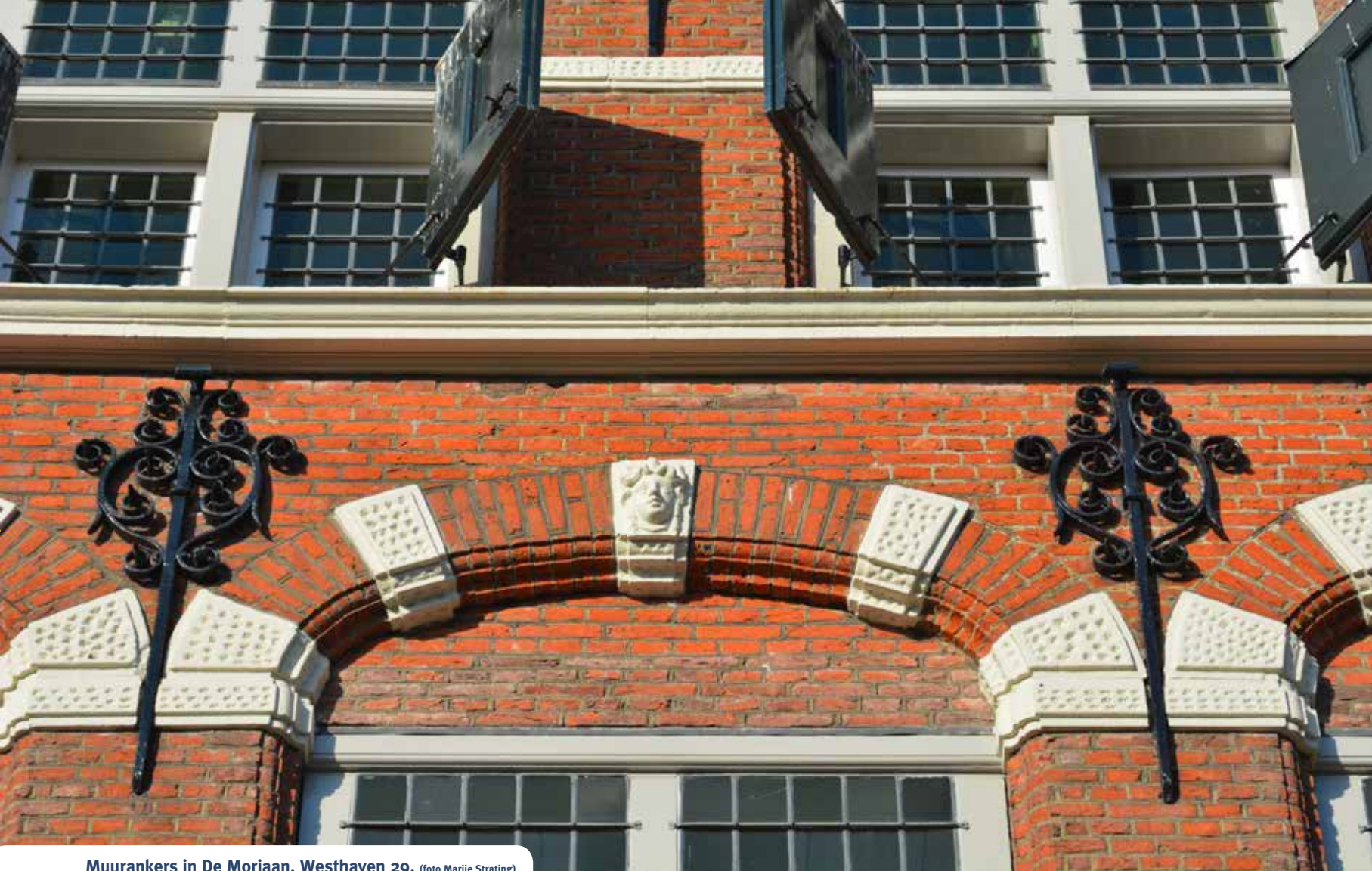
Muurankers in De Moriaan, Westhaven 29. (foto Marije Strating)
